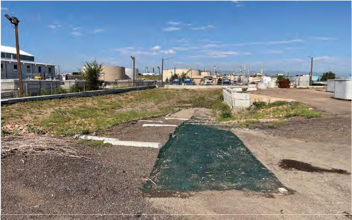
Photo 3 - A stormwater detention pond in the Project Area at 5901 Dexter Street
