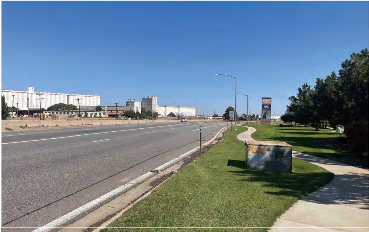
Photo 27 - Vasquez Boulevard facing north, toward the intersection with East 62nd Avenue
