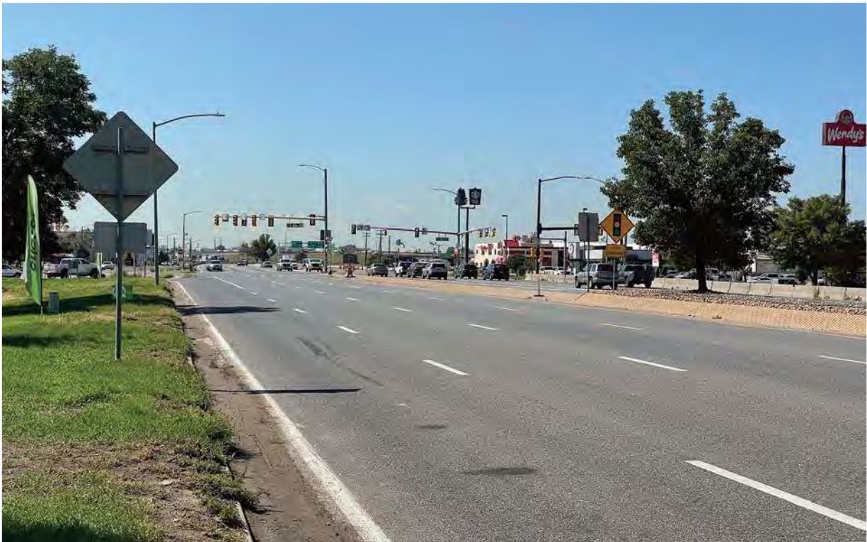
Photo 24 - Vasquez Boulevard facing south, toward the intersection with East 60th Avenue
