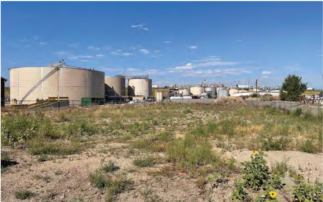
Photo 6 - The informal stormwater detention pond on the southwest portion of the Project Area
