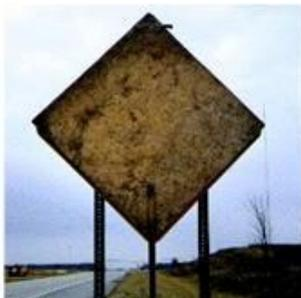
When signs are not in use, it is required that they be taken down or fully covered. Sign covers are detailed in the CDOT Specifications manual. Sign covers may be made of durable plastic, wood, metal, or polypropylene. Signs which are taken down or faced away from traffic, must be stored outside of the clear zone.
