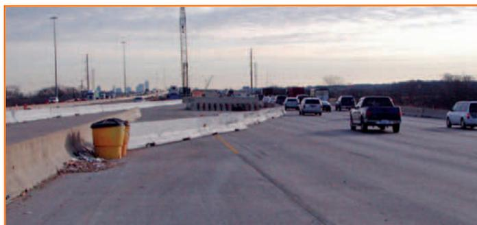
**Barrier ends in work zones must be protected by flaring them and/or providing crash cushions** (Source: TTI).
