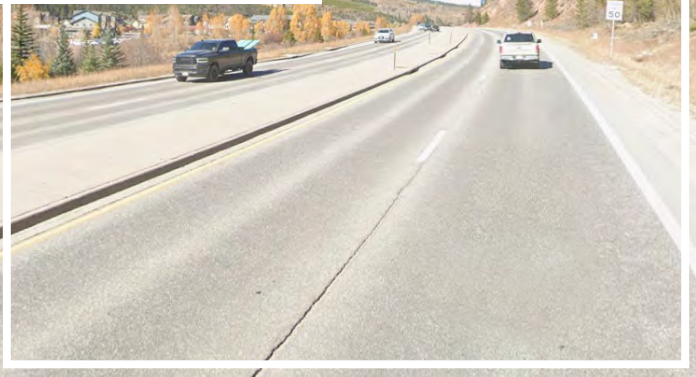
Rural Places Breckenridge, CO CO-9
