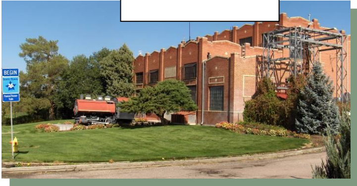
The skyline at Exit 80 is dominated by the grain elevators of the Great Western Sugar Company. This is the last large sugar-beet processing facility in Colorado. Could these structures, considered an eyesore by some, be used for a large-scale mural?
