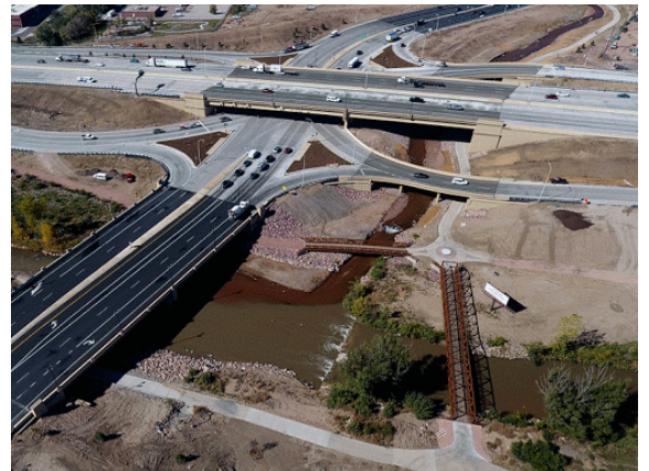
The new Cimarron interchange
