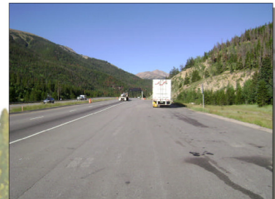
6. View west at truck chain up station Exit 228W
