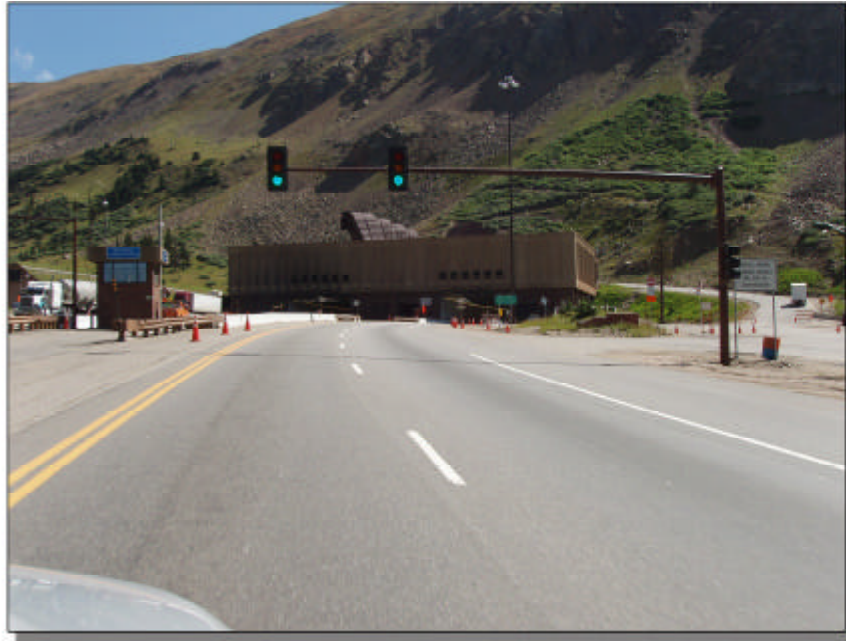
1. View of Eisenhower Tunnel, west portal
