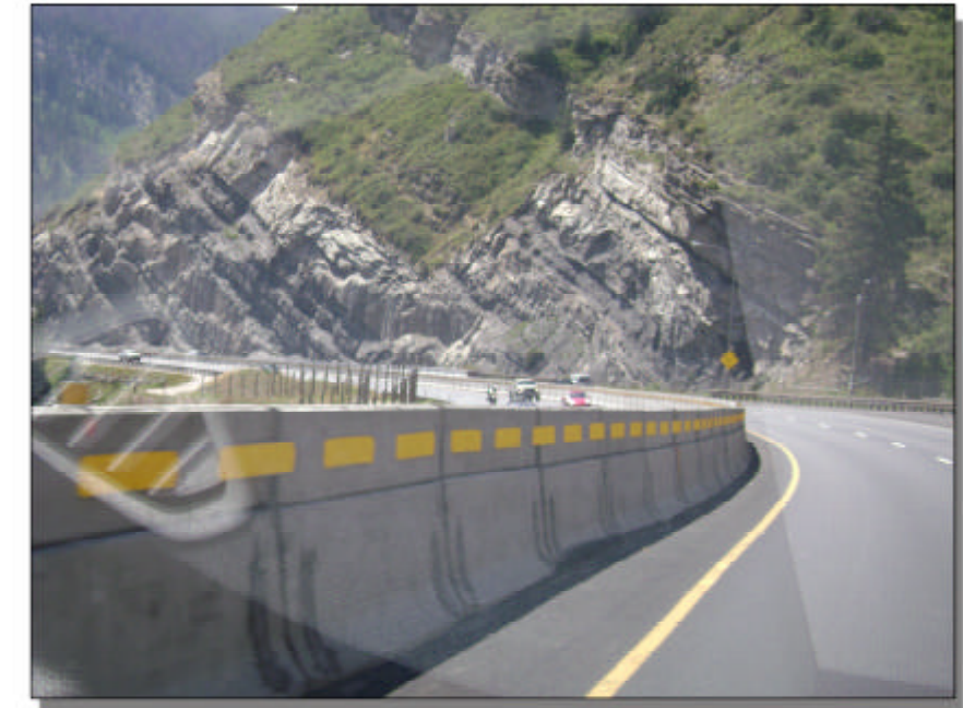
3. View west from Eisenhower Tunnel
