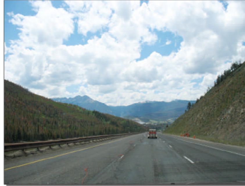
2. View west from Eisenhower Tunnel
