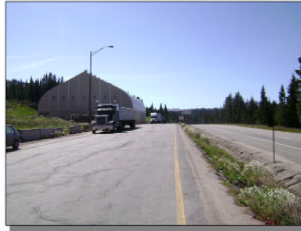
2. Vail Pass Maintenance Barn from west
