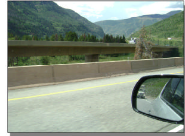
4. View west at bridges east of Vail
