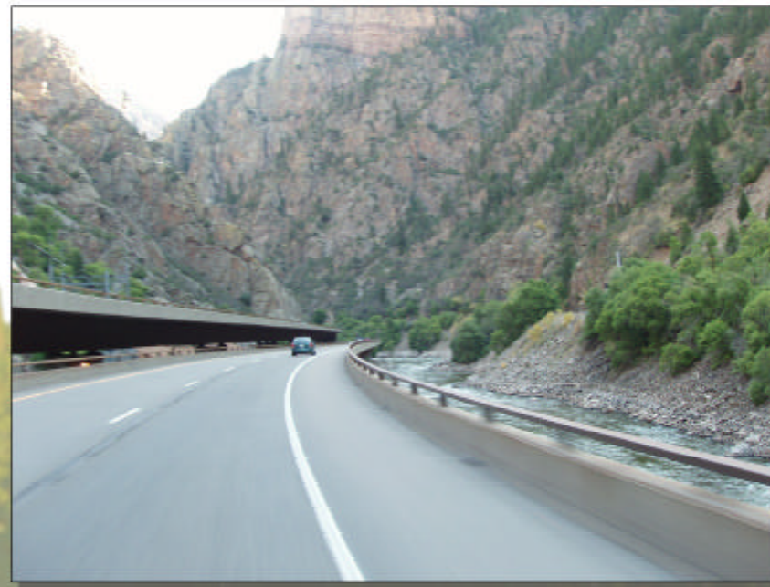
5. View west in Glenwood Canyon
