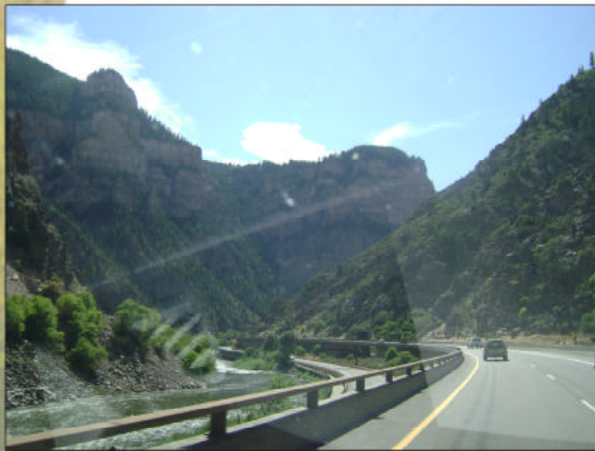
4. View west at entrance to Glenwood Canyon
