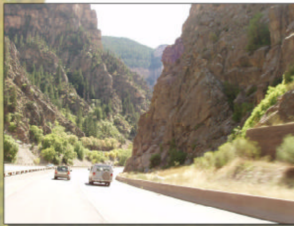
5. View west towards Glenwood Springs
