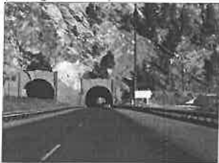
Existing Twin Tunnels (looking eastbound)
