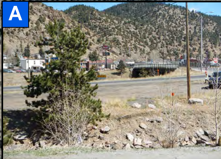
View of Chicago Creek Rd bridge and properties along Idaho St from south side of I-70
